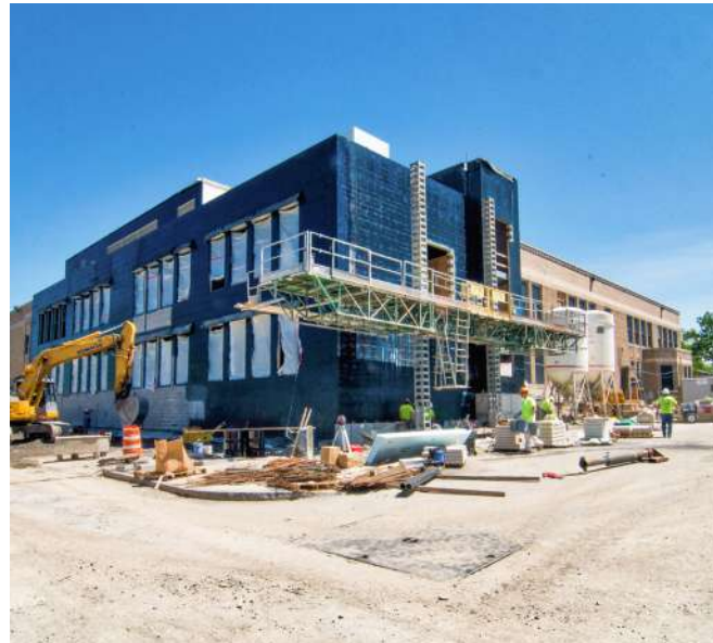
Construction of George Mather Forbes School 4
